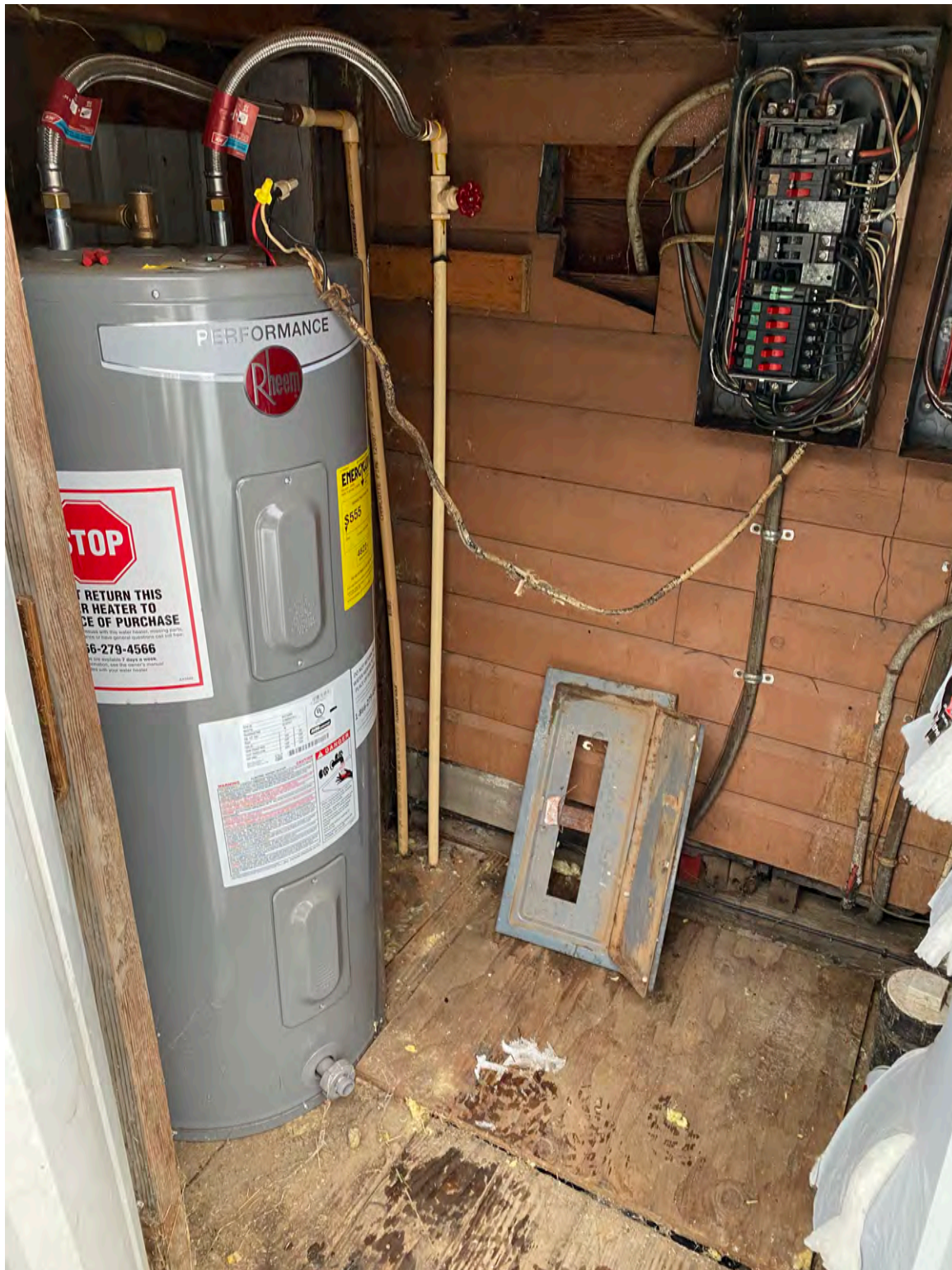
The electrical panels are indoor rated, affixed to the exterior of the building. The covers were in that position when we were called to the apartment. Also, notice the exposed wire nuts on the water heater.
